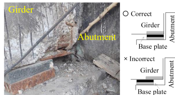
Figure 10 Deteriorations around the bearing
